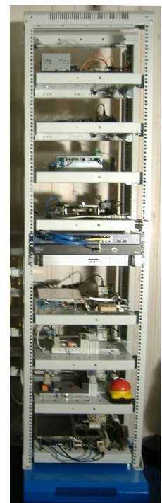
Figure 1: OSADL test rack
